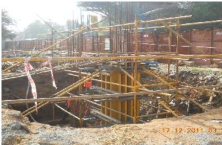
Column work at OTA station
