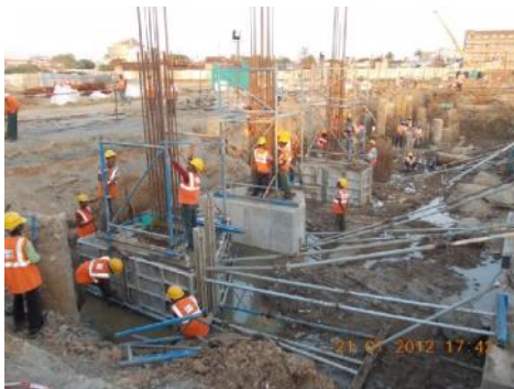
Depot administrative building work
