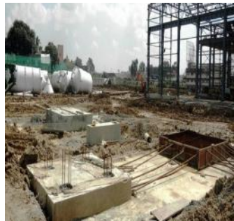
D wall auguring in process at KMC station
