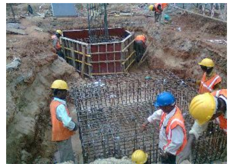
Pile cap reinforcement work at CMBT station
