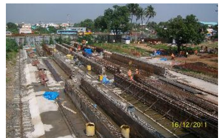
Precast girders at Vanagaram casting yard
