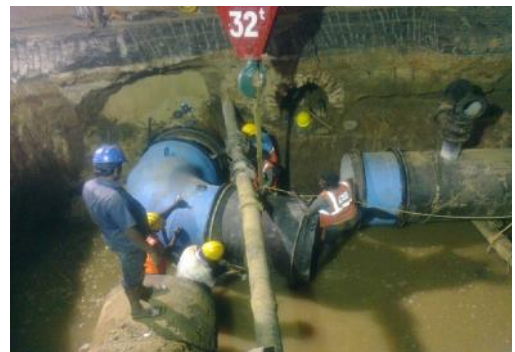
After diversion (Fixing of collar pipe)
