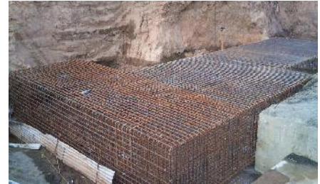
Footing reinforcement work at Ashok Nagar station
