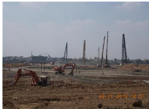
Earth filling and pile work at Depot
