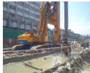
Cage lifting for D wall at Shenoy Nagar station
