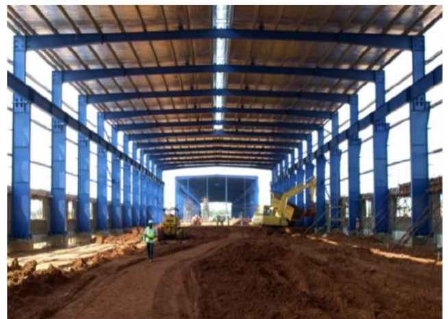
Fitting building work in progress
