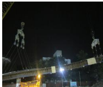
Cage lifting for D wall at Shenoy Nagar station
