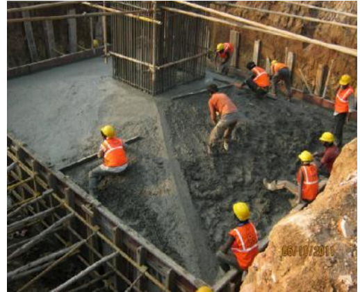
Tie beam work at Alandur station
