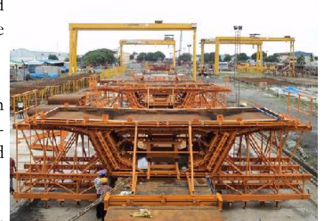
Form work for segment casting
