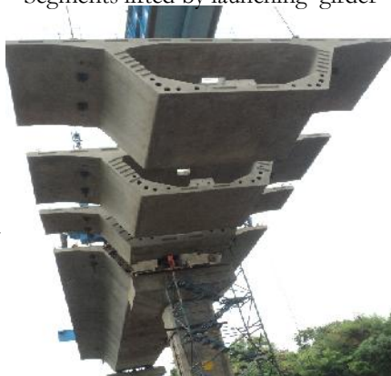
Segments lifted by launching girder
