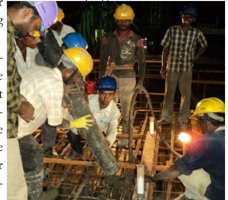
Pumping of concrete
