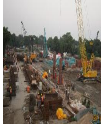
Work in progress at Washermenpet station
