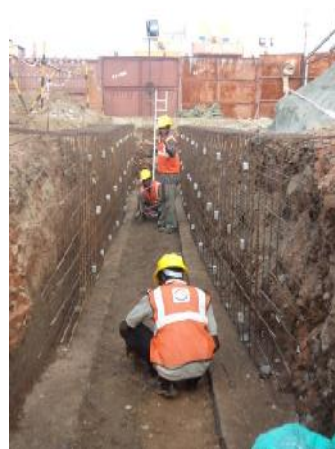
Guide Wall Work at Central
