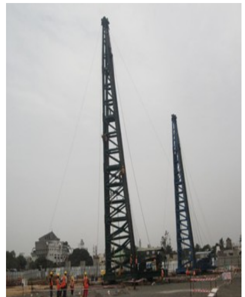
Pile rig work depot site
