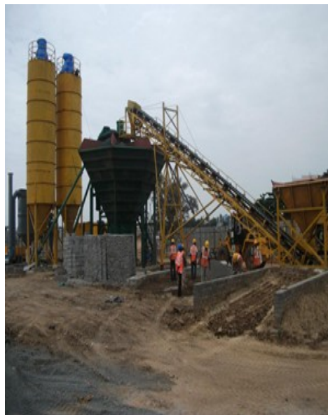
Batching plant work depot site
