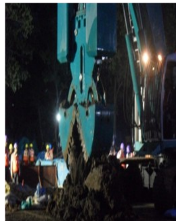
Diaphragm wall work at Washermanpet station
