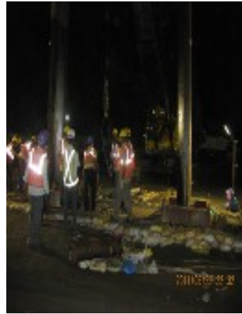
Diaphragm wall excavation at Shenoy Nagar station
