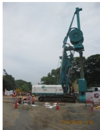
Diaphragm wall work at Washermanpet station
